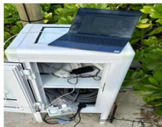
Cable and power system located at the beach. Cables go from the beach to the camera underwater to supply power to the camera.
